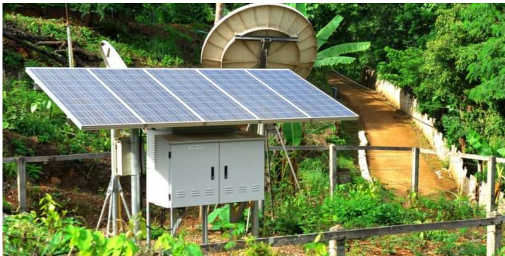
Figure 2: Off-grid solar system (Photo from Afrik21 2020)
